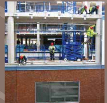
Fixing of external cladding panels
